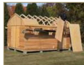
Roof trusses and sheathing is installed
