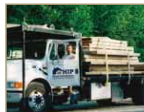
Truck arrives with prefabricated shed sections
