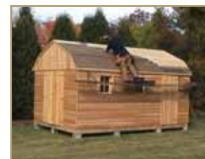
Roof shingles are applied
