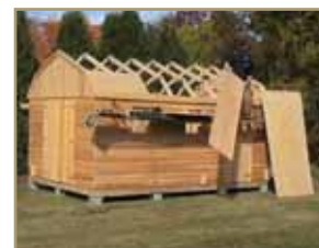
Roof trusses and sheathing is installed
