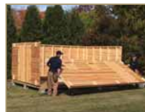
Wall sections are positioned and nailed into place
