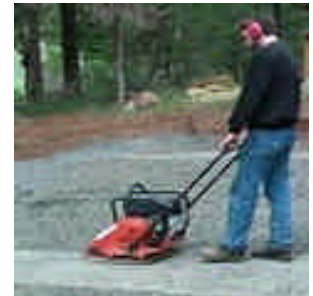
Using a plate compactor to pack the gravel
