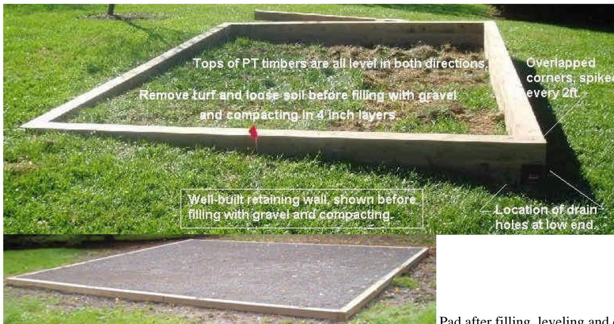
Pad after filling, leveling and compaction.
