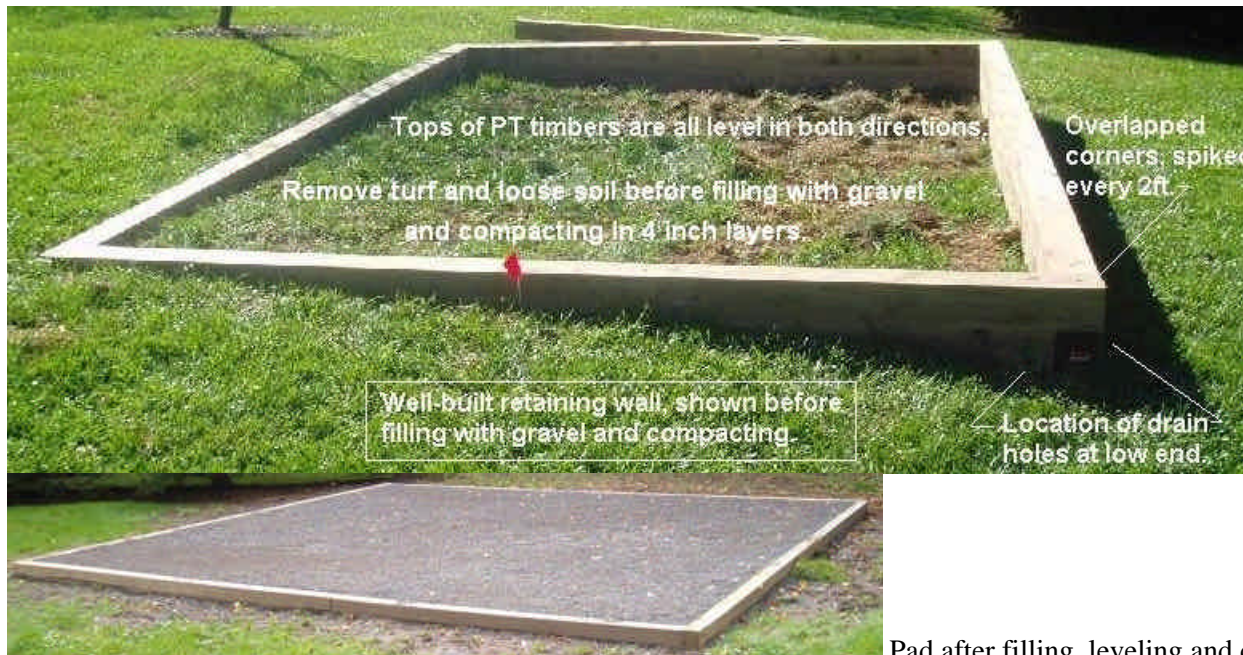
Pad after filling, leveling and compaction.
